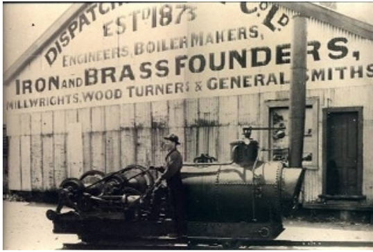
An early photo of the Dispatch Foundry and a steam log winch which is being used as a model for the created foundry.
