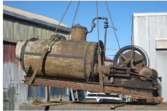
Restoration of the Steam Log Winch at Dispatch Foundry.
